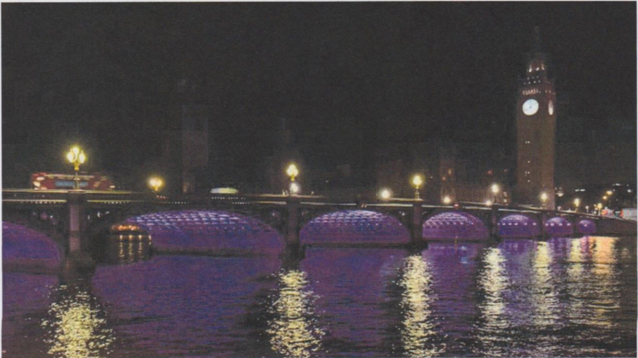
Illuminated River on Westminster Bridge - ©Paul Crawley
