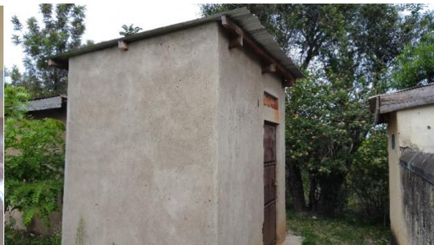
Changing room built in Nambogo primary school
