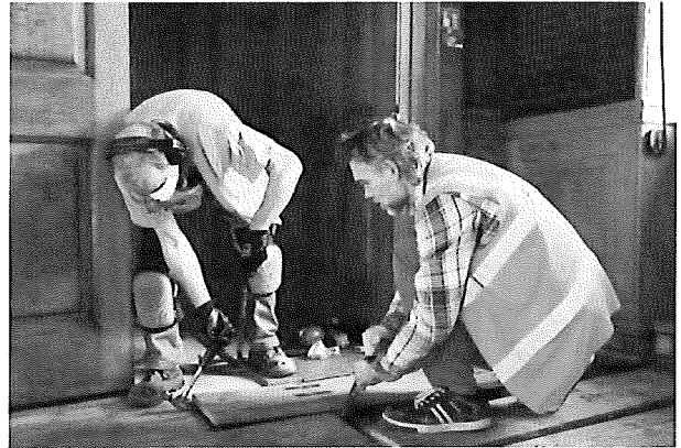
Work begins on lifting the floor of the Great Hall to allow new services to be installed (Photo: Matthew Andrews)
