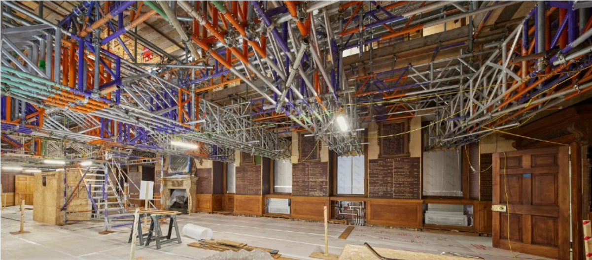
The 'bird cage' scaffolding in the Great Hall (Matthew Andrews)
