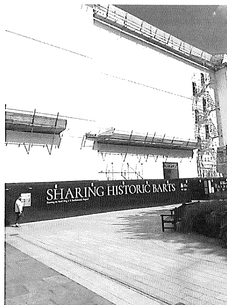
The North Wing, under scaffolding, April 2024
