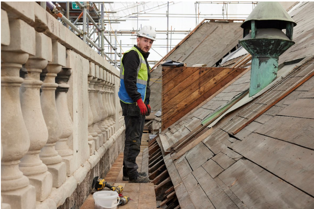
Repair works to North Wing roof in progress (Matthew Andrews)
