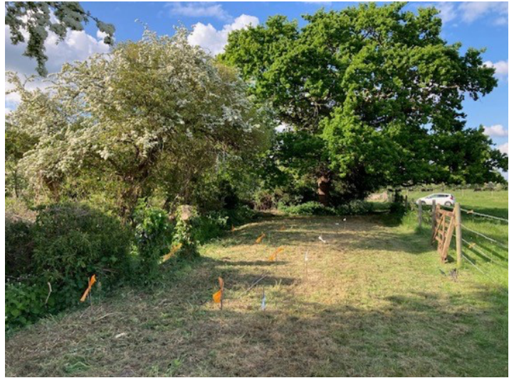
Setting out of the eco-toilets' footprint in early May
