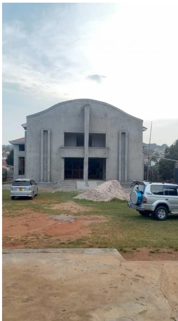
1 Progress on church building in Uganda.
