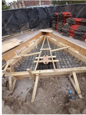
Securing the foundation
