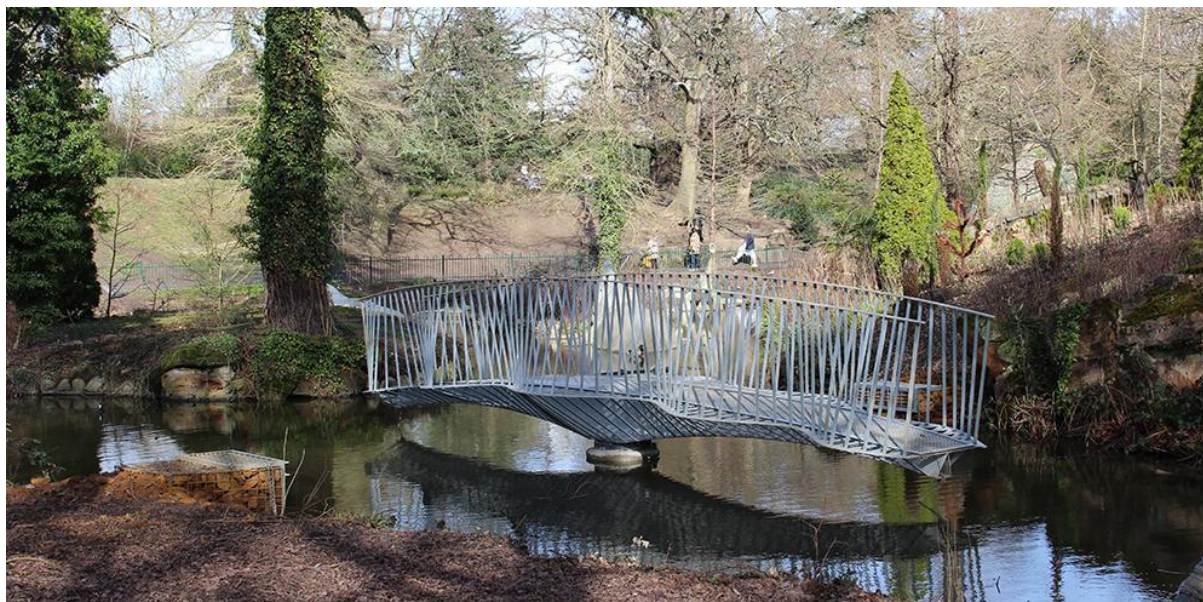
The bridge shown rotated to the locked position. © Friends of Crystal Palace Dinosaurs
