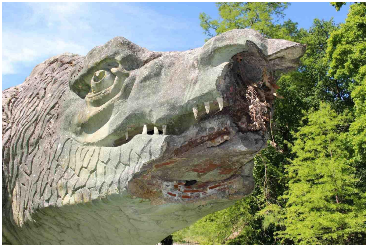
Detail of the damage to the Megalosaurus jaw showing exposed concrete, iron structural support and brickwork. © Friends of Crystal Palace Dinosaurs
