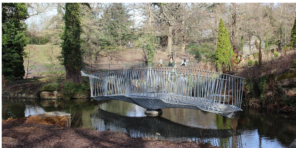
Figure 8: The bridge shown rotated to the locked position, preventing unauthorised access to the Dinosaur Islands. © Friends of Crystal Palace Dinosaurs
