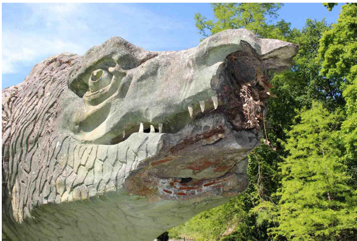
Figure 1: Detail of the damage to the Megalosaurus jaw showing exposed concrete, iron structural support and brickwork. © Friends of Crystal Palace Dinosaurs
