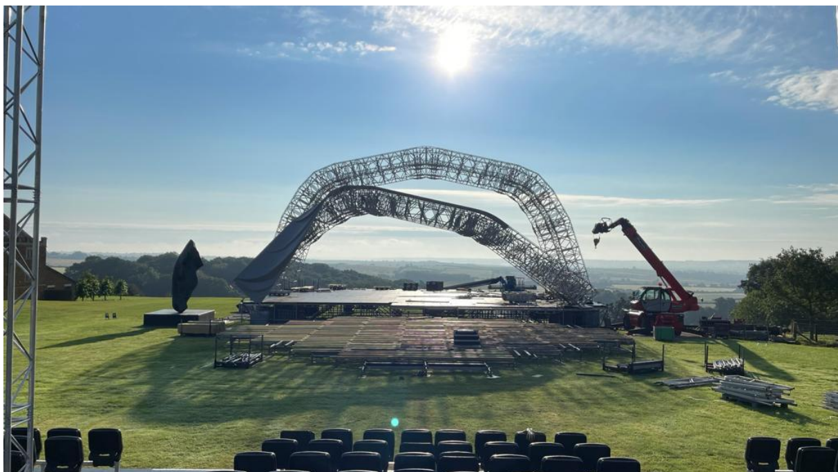
Construction began for the temporary theatre at Nevill Holt, summer 2021
