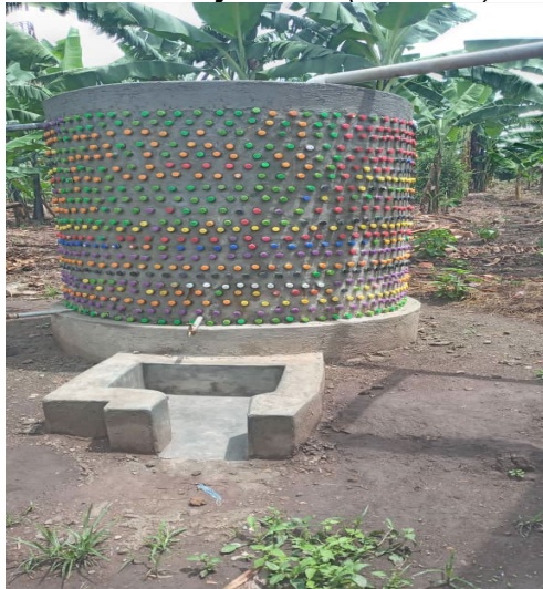
Water Tank built with Empty bottles
