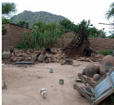
The fallen building
