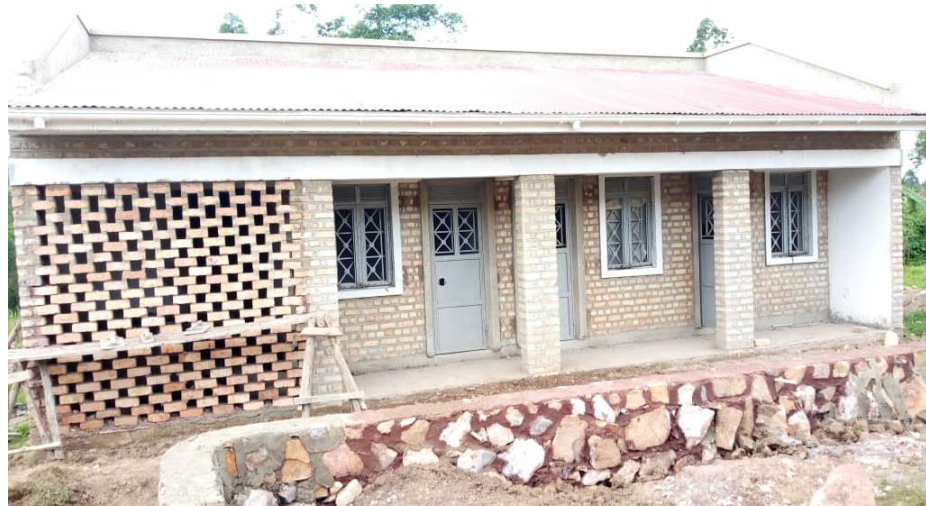
Staff house and outside kitchen
