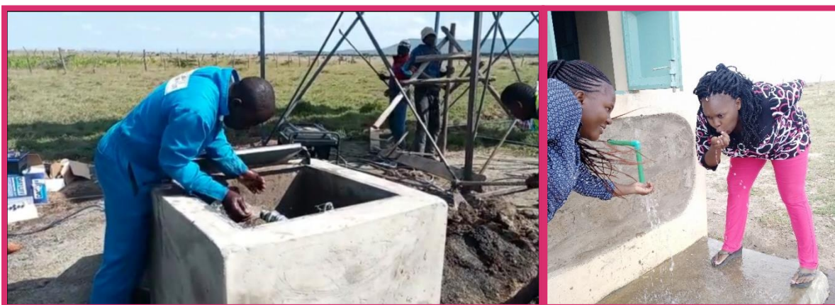
1. Installing the water solution
