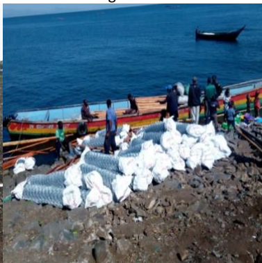
Fencing materials arrive
