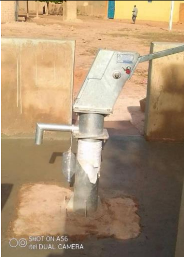
Water wells drilling
