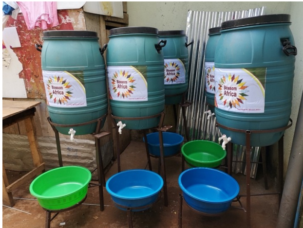
Handwashing facilities for the resettled community
