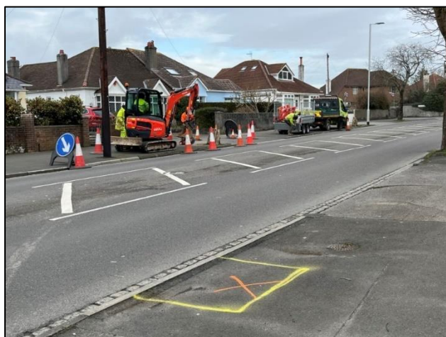
Glendale Countryside on Beacon Park Road, 27 th February 2024
