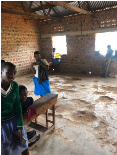
Classrooms before floor cementing
