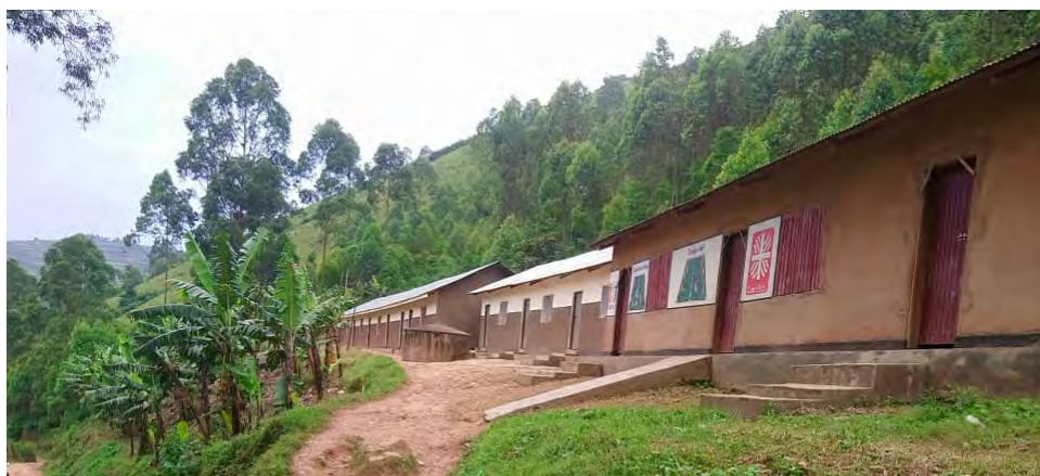
Kyeibale Primary School has been completely rebuilt following a landslide
