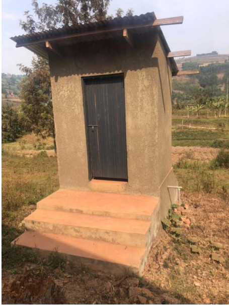
Kanjobe Primary School Ecosan latrine
