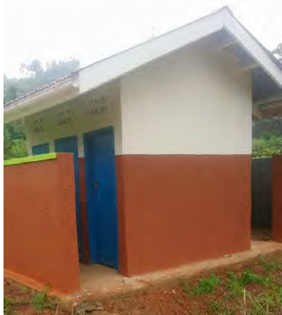
Kamuronko School latrine
