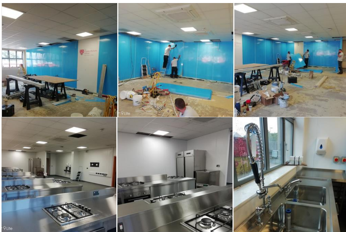
Preparation work and completed Food Technology Room – The Charles Dickens School
