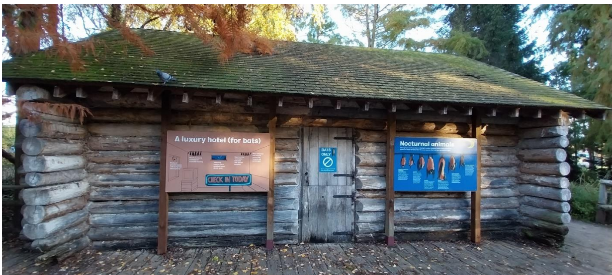
Newly modified "bat lodge" at WWT London Wetland Centre
