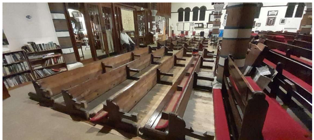
Neil Woolley pauses for a rest after safely completing stage one of the pew removal
