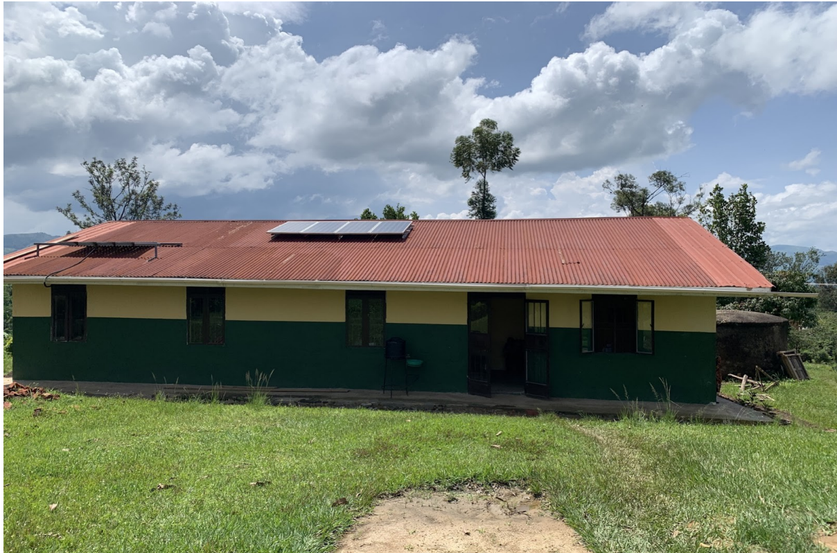
Outside of the health centre on completion of the renovation project.
