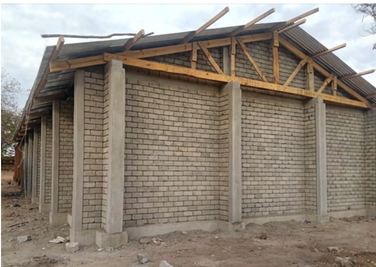
The roof going on and the completed classroom
