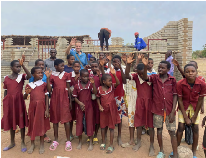
Nkhwikwi school under construction October 2024.
