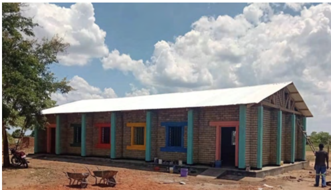
Nkhwikwi school block just completed
