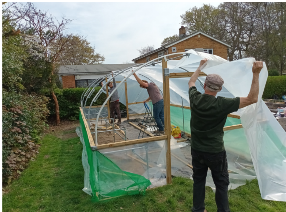
Fig 1 – Installation of the new poly tunnel at Pelhams Park
