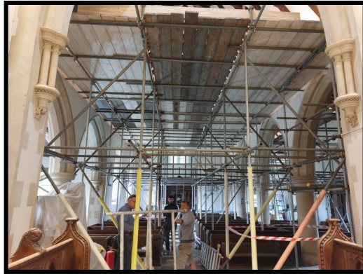
Scaffolding towers during the re-decoration in 2024
