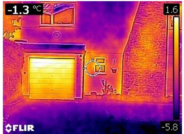
Thermal image of a local home. The yellow shows the warmer areas which may be sources of heat loss.
