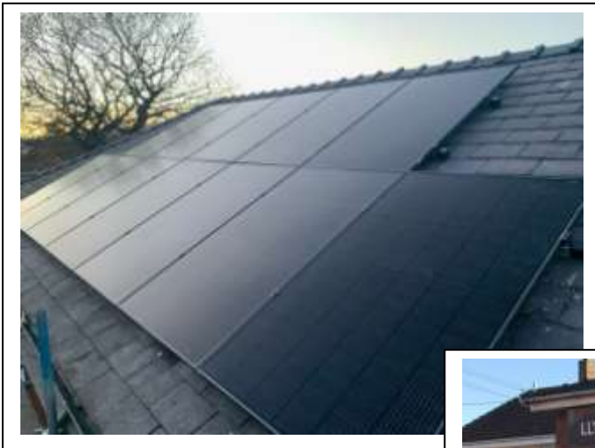
Solar panels going up, and our lovely new sign
