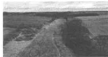
View of top section of site before works Credit: Andrew Chick
