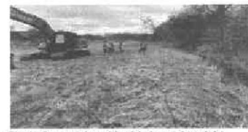
Site before works with old channel to right Credit: EA
