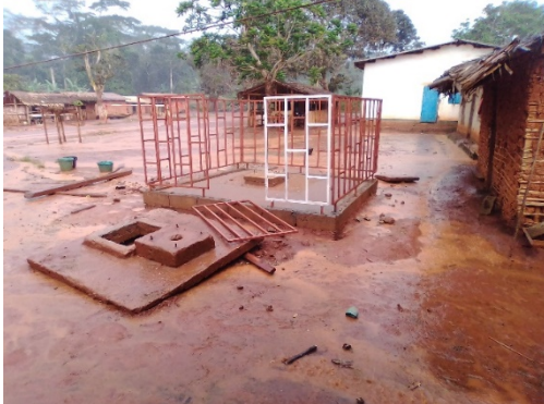
Photo 2: KASSARAFAM Village during the works
