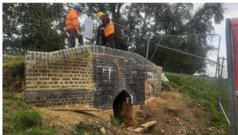
Above left rewatering section 2 towards the oil pipeline crossing Above right rebuild flood sluice near bridge two
