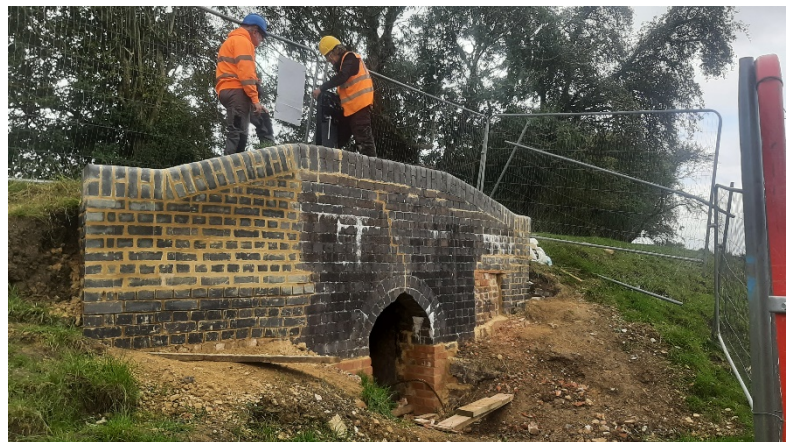
Above left rewatering section 2 towards the oil pipeline crossing Above right rebuild flood sluice near bridge two
