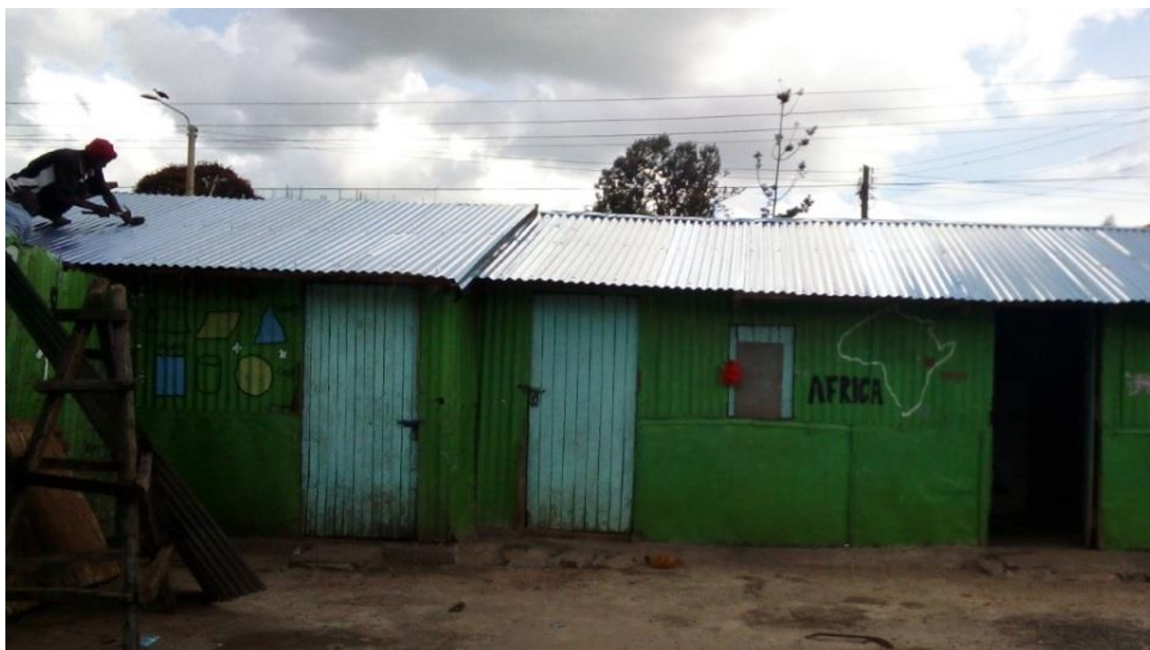
Figure 9: New roof at Excel
