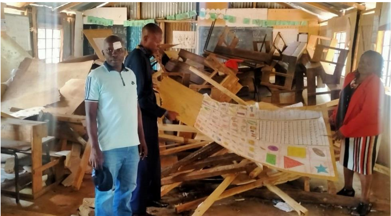
Figure 12: Damage at Compassion School
