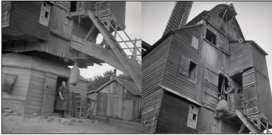
The Rex Wailes Collection is a rich resource for mill researchers both in the UK and around the world. This pair of recently scanned images shows the miller and his wife operating the sack hoist at their mill, Moulin Deschodt, Wormhoudt, Nord, France ca 1950.
