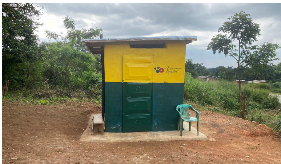
Latrine in Petit Bello
