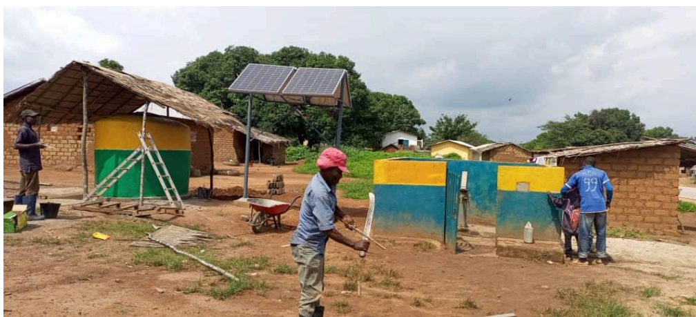
Solar Pump Retrofit in Mbangué
