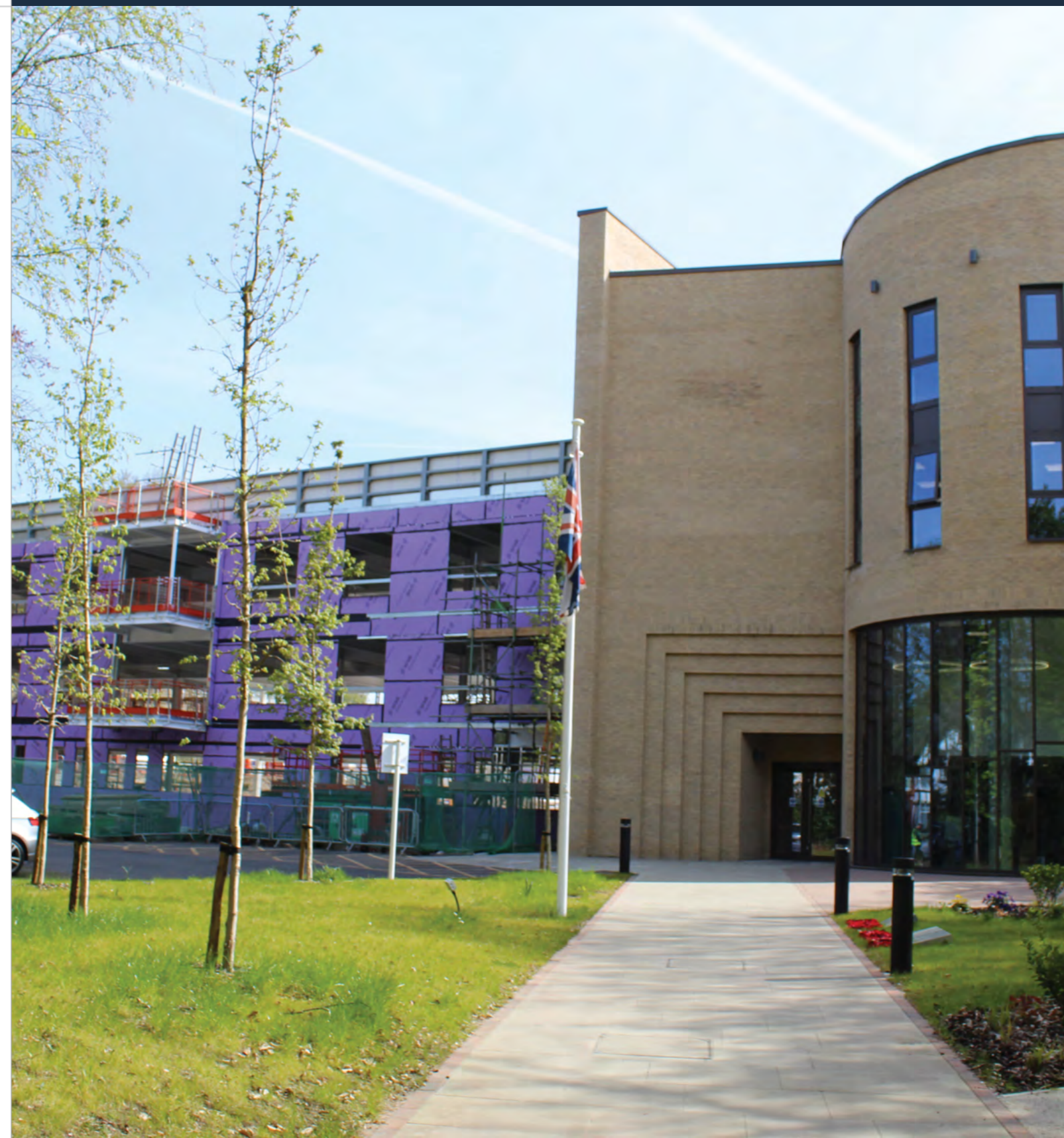
BROUGHTON HOUSE - VETERAN CARE VILLAGE PHASE 1B UNDER CONSTRUCTION
