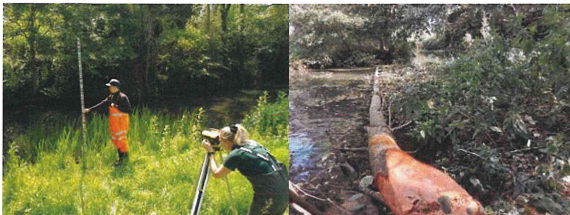
Image: the BART team undertaking a detailed site survey, and on the right, a hinged tree installed on the Sherston Avon, to improve flow diversity and habitat to support wildlife
