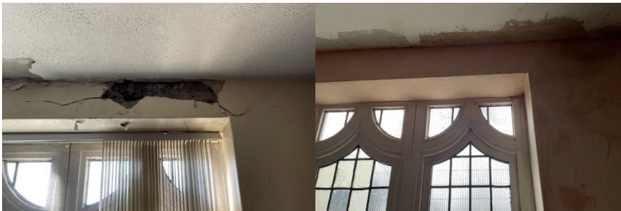
All Saints repair to ceiling (Choir Vestry )Before and After
