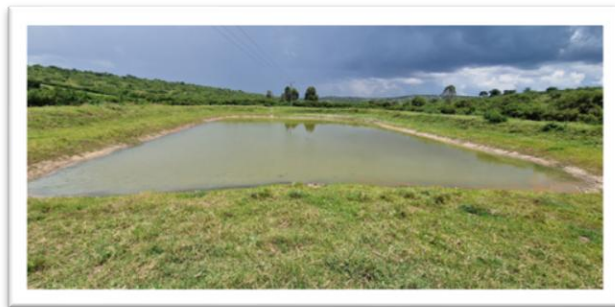
Valley tank well looked after by the community, November 2024.
