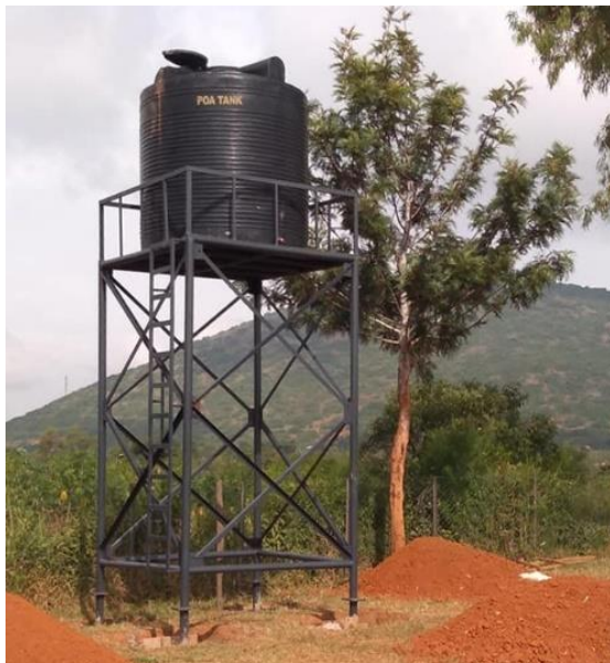
Figure 10: The new water tower
