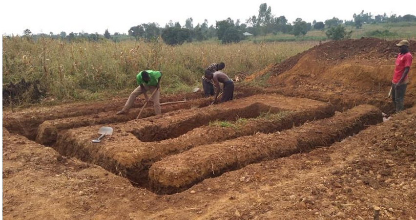
Figure 11: Toilets being constructed
