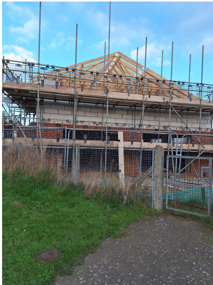
Roof Trusses in place and walls nearly complete in November 2025
