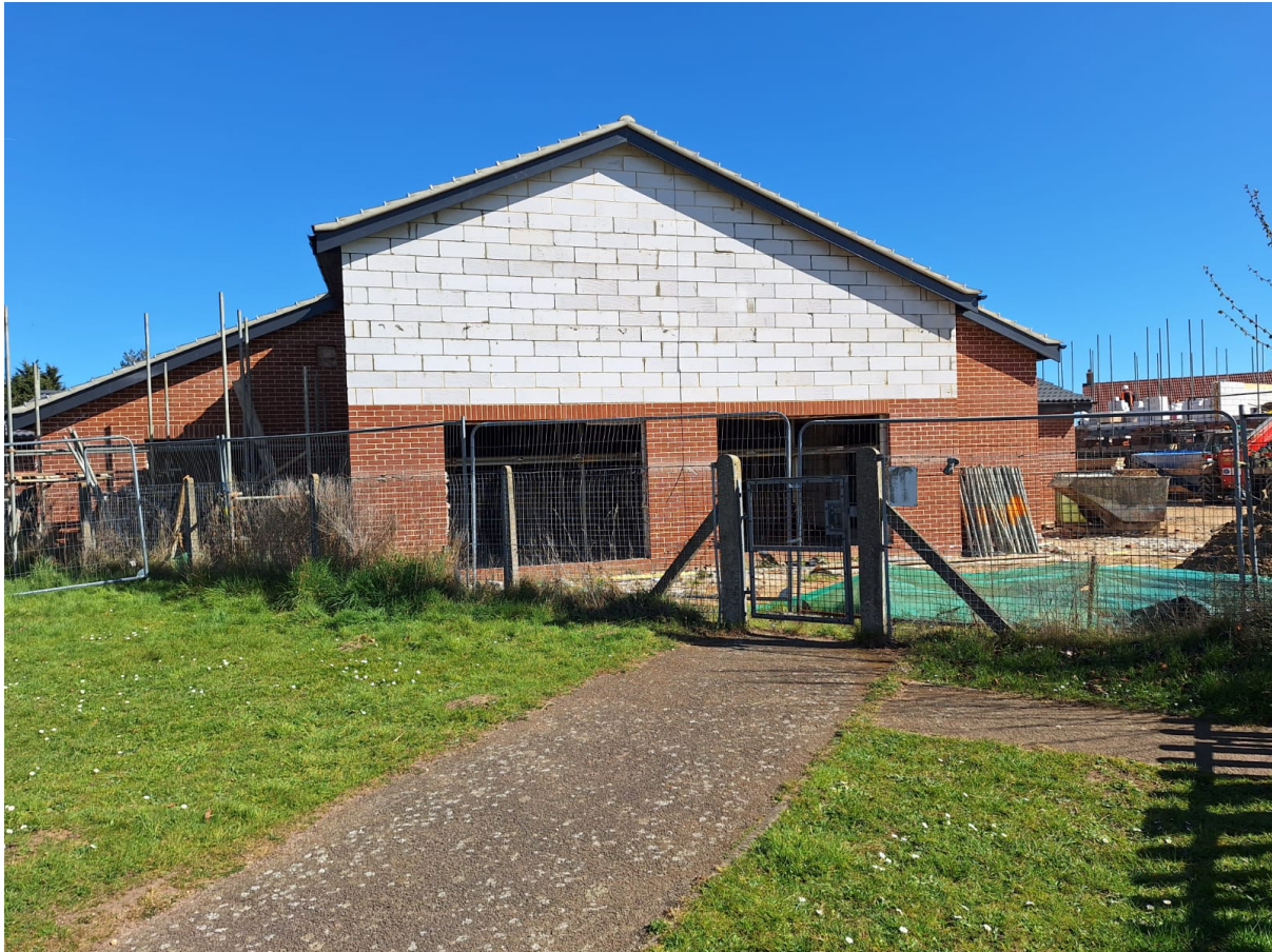
Building with tiled roof awaiting doors and windows to be fitted
