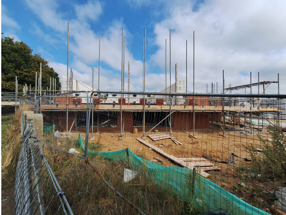
Construction of the walls well underway in September
