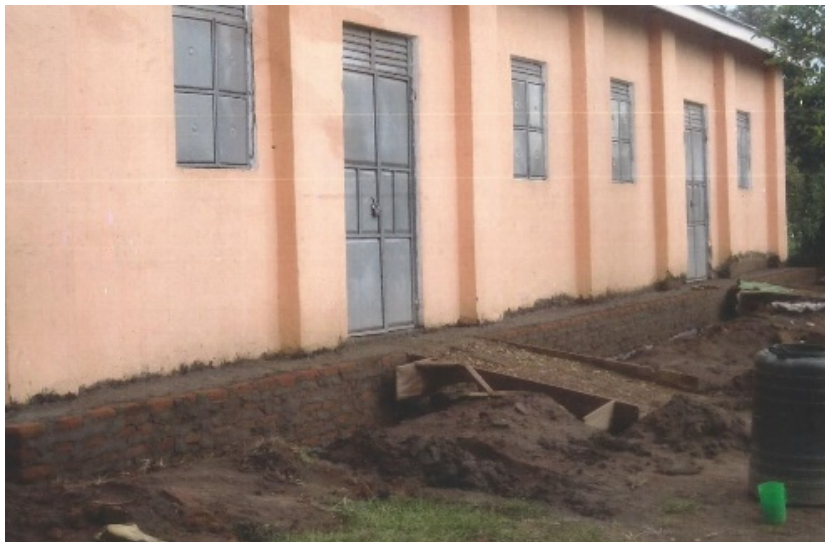
Veranda & disabled access to main Lwanjinsi site entrance
