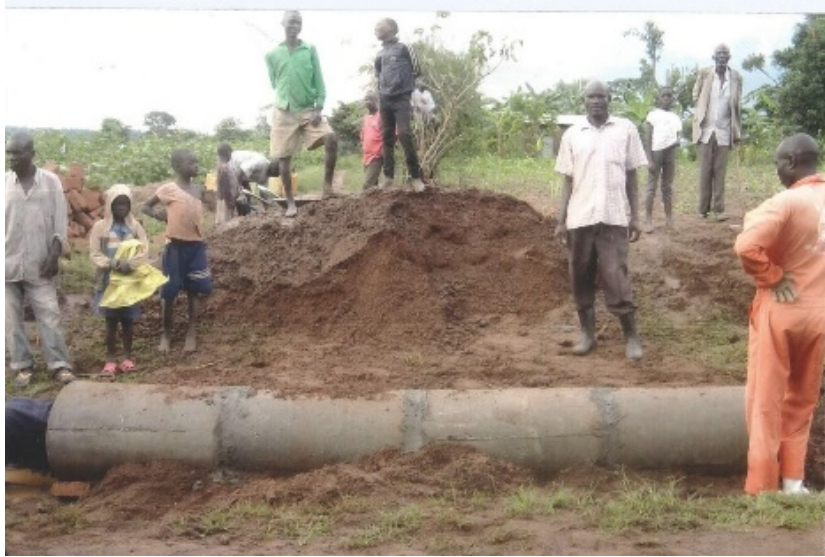
Provision of Rainwater culvert
