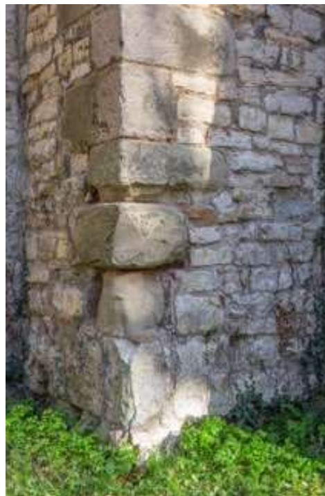
Erosion allowing Water Ingress
