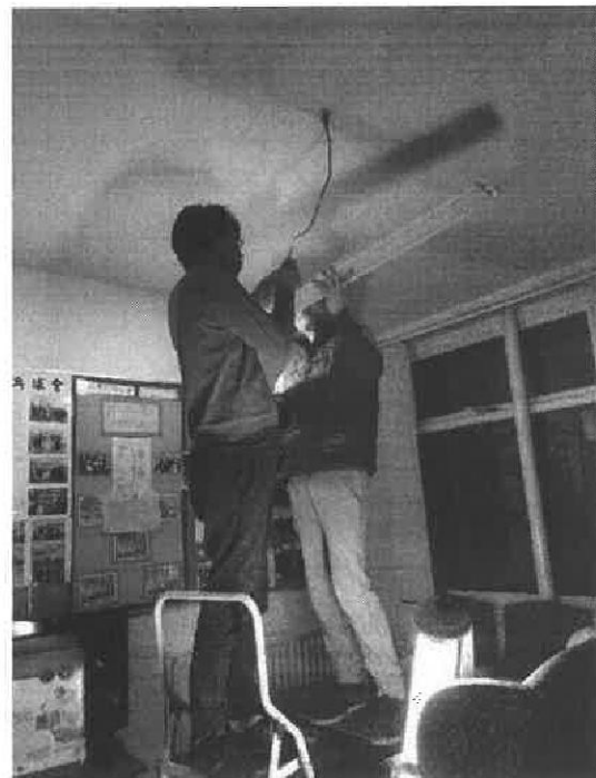
Volunteers helped to install LED lightings for the Centre
