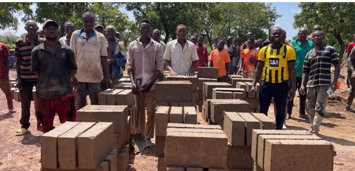
Parents of Tuopare JHS students building the new school kitchen
