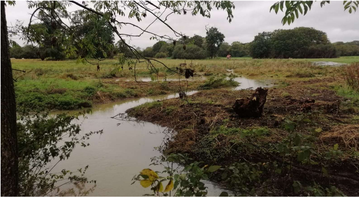
Natural Flood Management work in Gissing – reinstatement of an old paleo-channel
