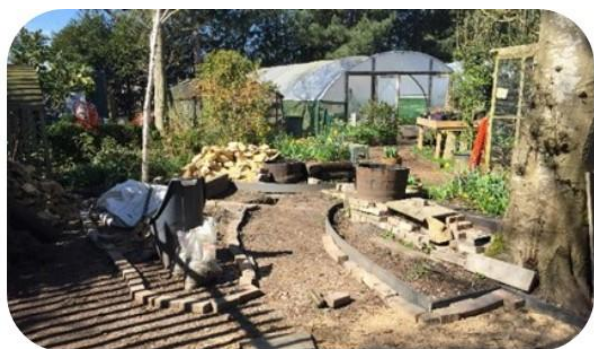
The Garden of Hope under construction.
