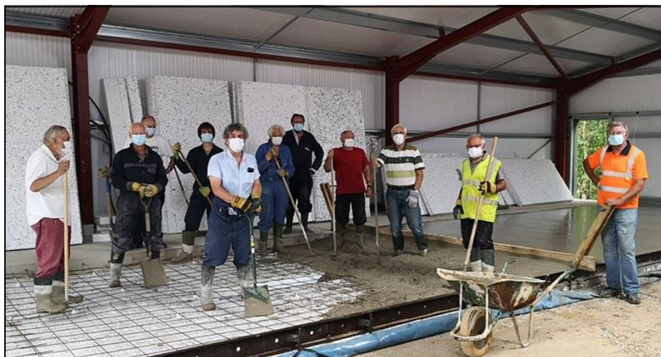
Construction work in progress with GHC members laying the concrete floor.
