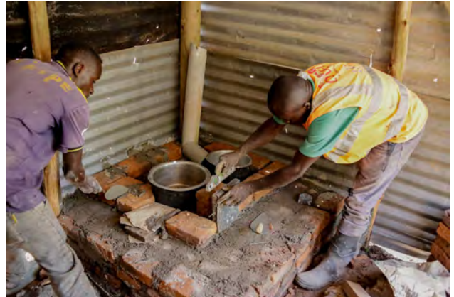
K4C Builder (Peter) constructing a new Lorena Stove for a family in Fort Portal (Uganda)
