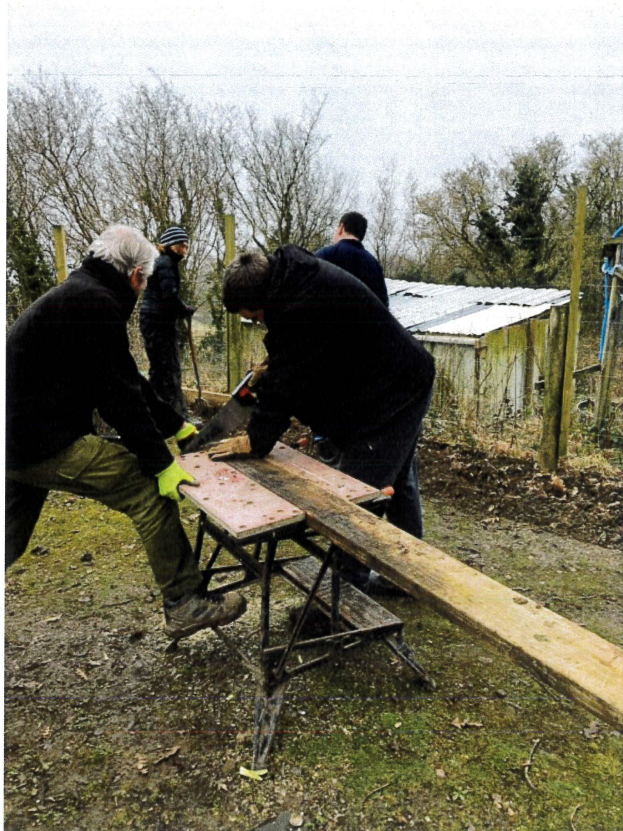
Volunteers working together to build new raised beds
