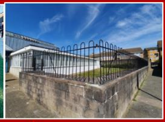
SACRISTY RENOVATION + HOT WATER
