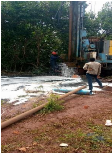
Asossa water supply deep well drilling.
