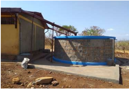
Roof water harvesting structure (Abora)
